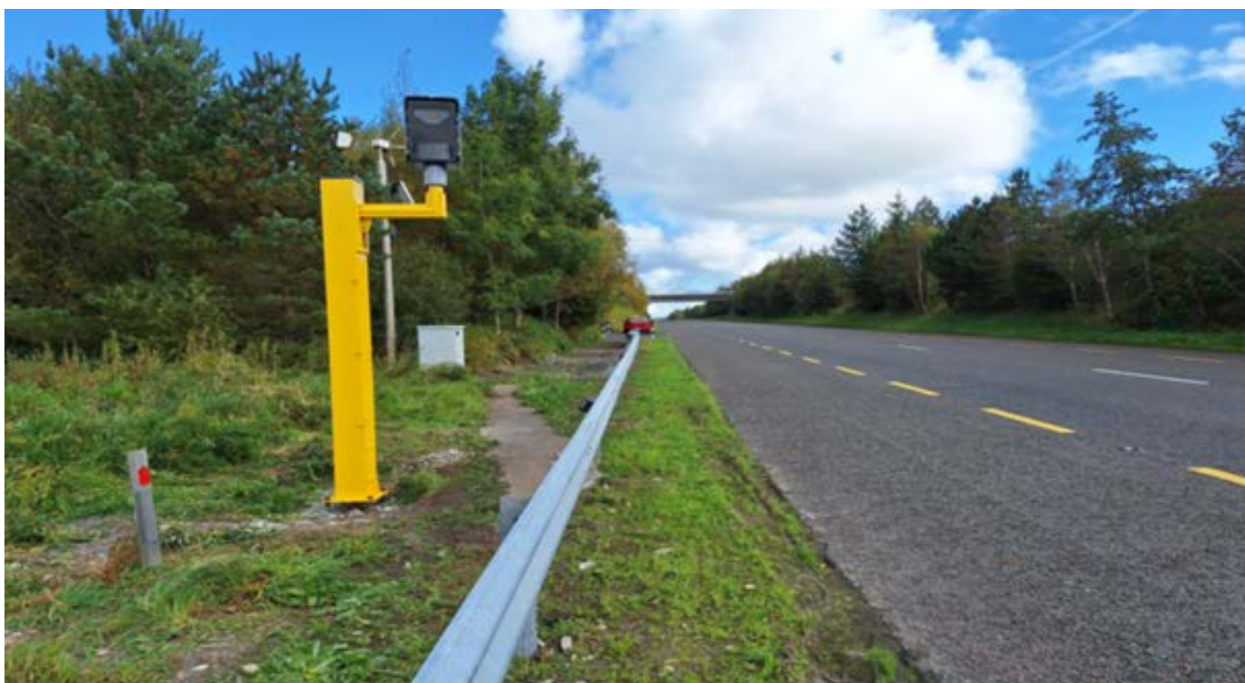
Image: N5 average safety camera (testing) Co. Mayo September 2024.
