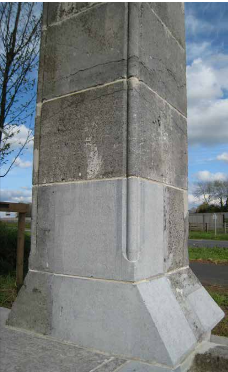
Detail of column stone restoration.
