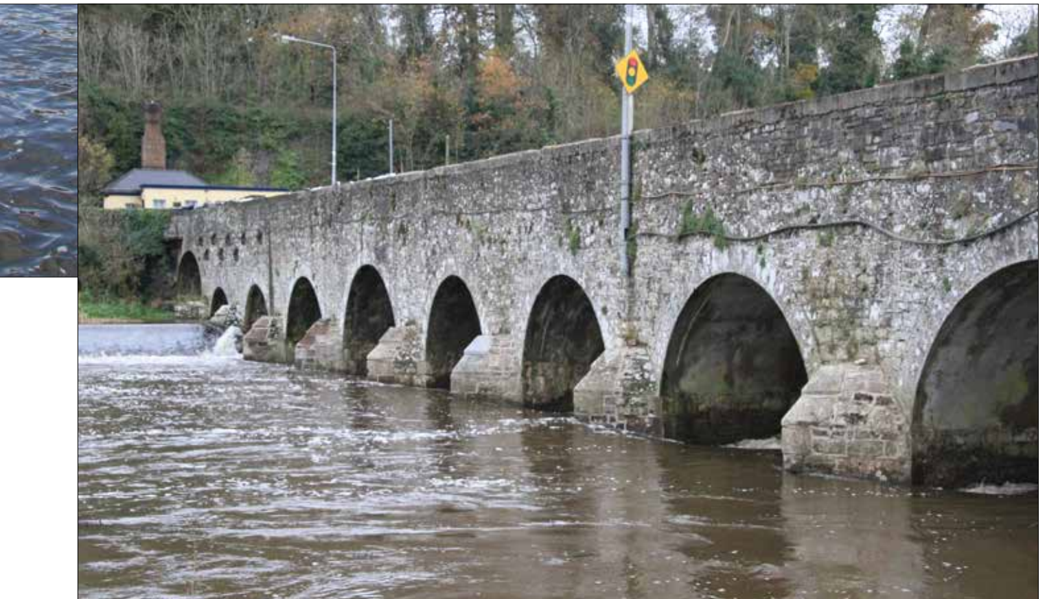
Eighteenth-century round arches on upstream side of bridge.
