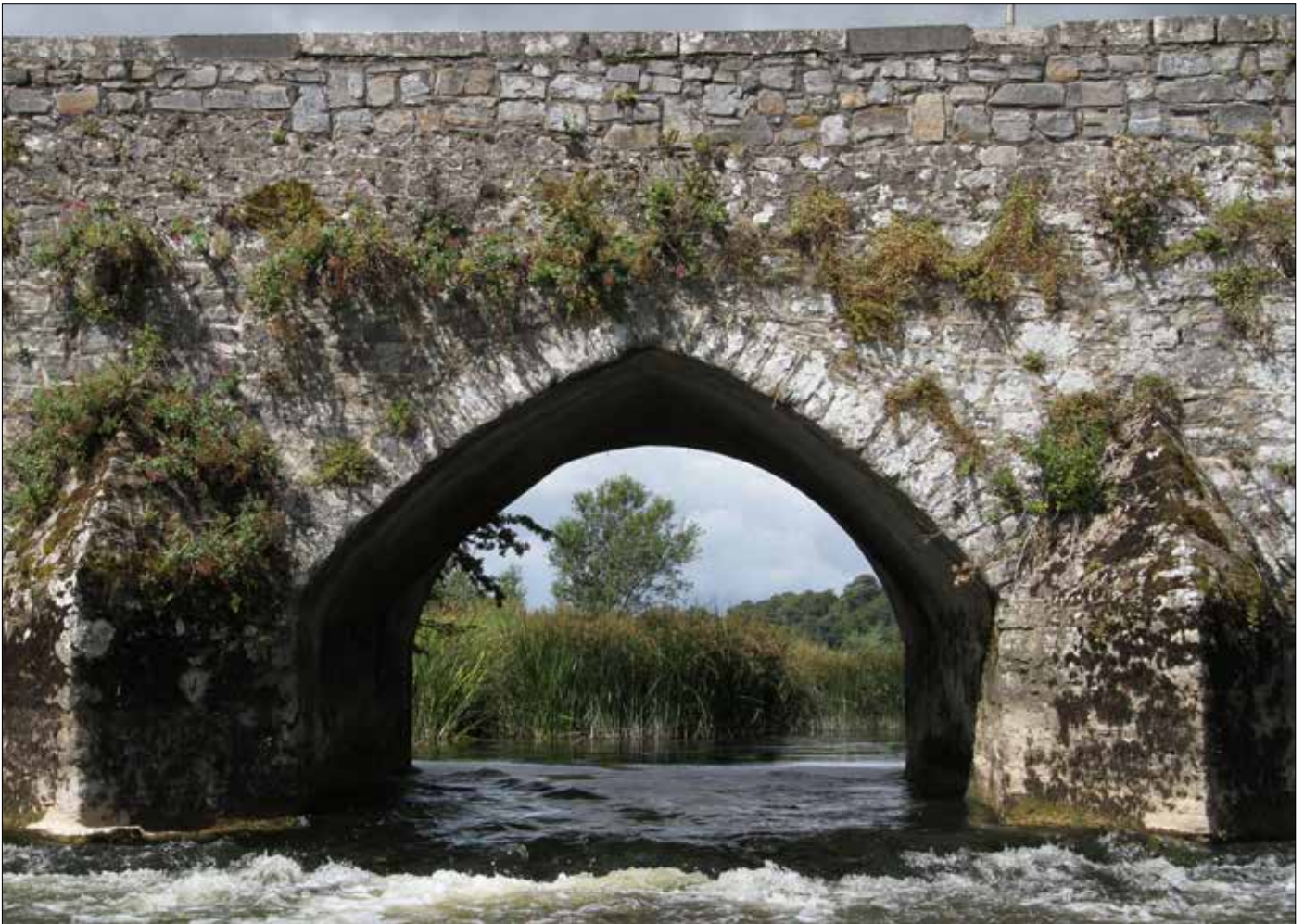
Medieval pointed arch, with 18th-century round arch at rear.
