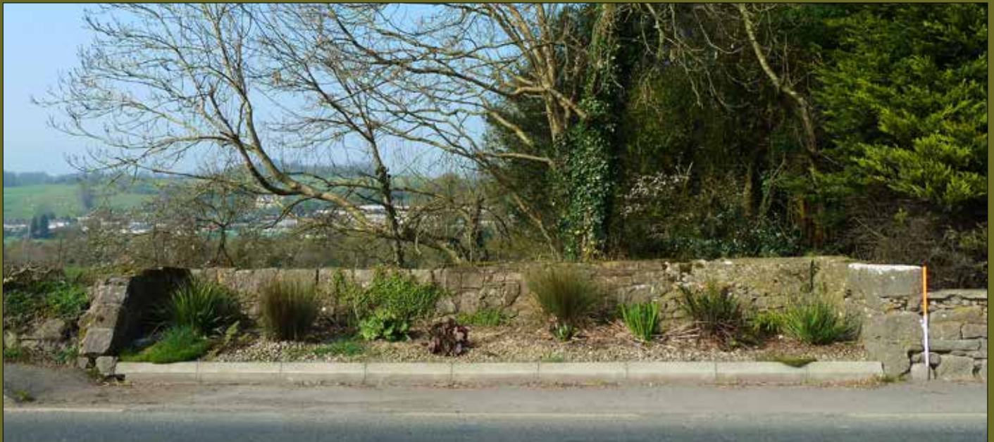
A stone depot on the N72 near Cappoquin. (Photo: Bernice Kelly)
